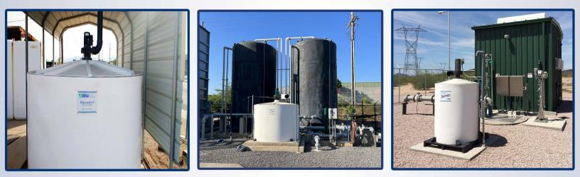
•Peacemaker<sup>®</sup> Scrubbers with Peacemaker<sup>®</sup> Converting Media: Removes H2S loading's greater than 2000 PPM.
