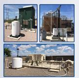
PEACEMAKER® Dry Air Scrubbers can be used as a single vessel, two vessels in series, or two vessels in parallel. The scrubbers provide two stages of media for the control of hydrogen sulfide (H2S), and other odors generated in wastewater collection systems, manholes and lift stations along with controlling various point source odors present in wastewater treatment plants. Our scrubbers are maintenance free, effective, economic and require no water addition.
