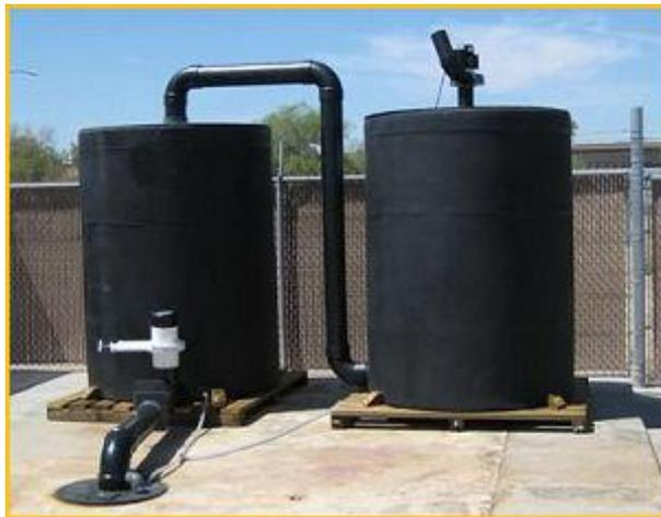
**How much airflow is required?** Benefits accrue from moving only enough air to maintain a slight negative pressure. This will prevent fugitive malodors and provide the best economics. Higher-than-necessary airflow increases static pressure through the media bed and reduces residence time. A larger scrubber may be needed and cost would increase.
