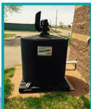
**PEACEMAKER® Dry Air Scrubbers** Are used as a single vessel, two vessels in series or two vessels in parallel. The scrubbers provide two stages of media for the control of hydrogen sulfide ( $H_2S$ ), and other odors generated in wastewater collection systems, manholes and lift stations along with controlling various point source odors present in wastewater treatment plants. Our scrubbers are maintenance free, effective, economic and require no chemical addition.
